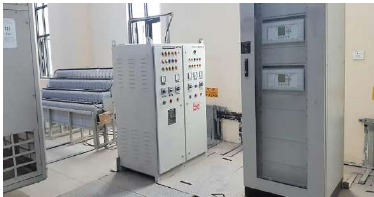
SCADA RTU Panel in Metro Station
