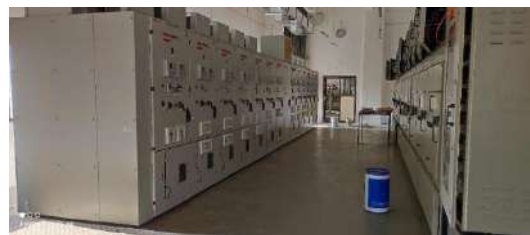
33kV & 25kV Switchboards in Range Hill RSS
