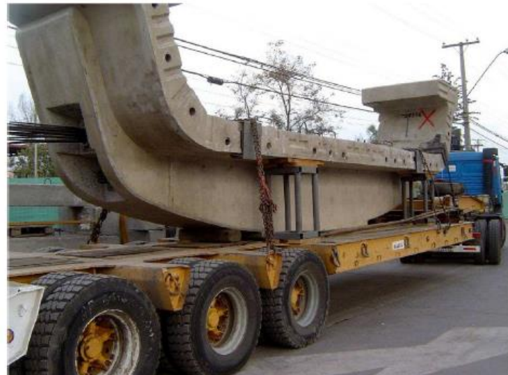
Figure 64 : Transporting of Precast Segments from precast yard
