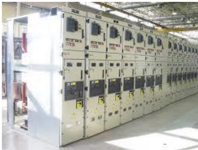
Figure 108 : Typical Indoor Auxiliary Sub-station
