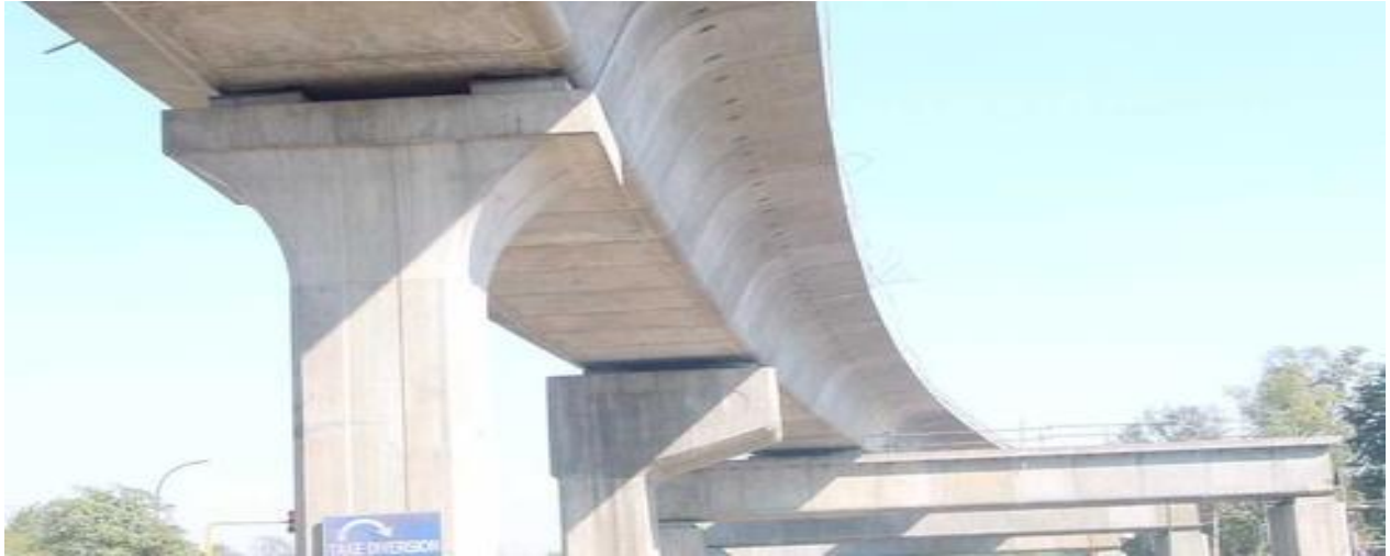
Figure 58 : RC Pier cap for Segmental Box-Girder Viaduct
