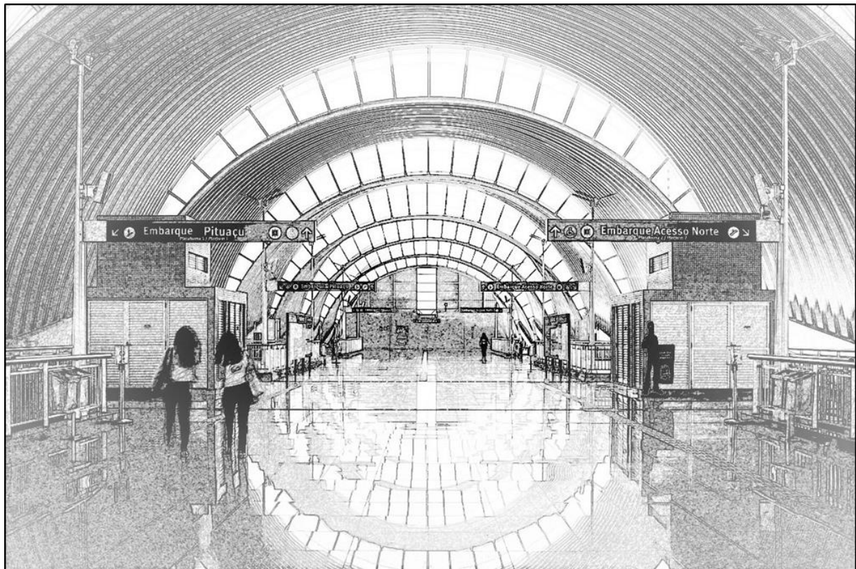
Figure 94 : Glasses used for natural light from sides and Skylight from roof
