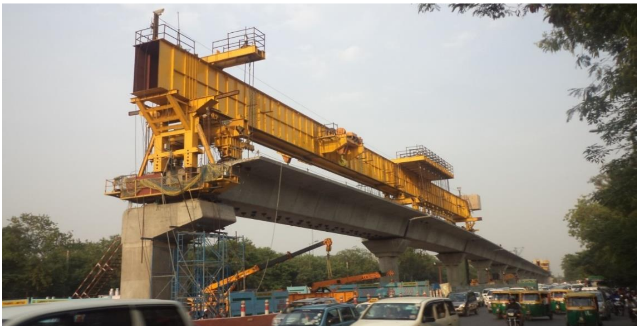
Figure 60 : Launching Girder – Precast segmental Box Girder Construction
