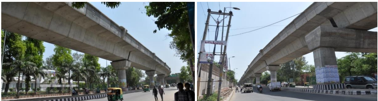
Figure 57 : Precast Segmental Box-Girder Viaduct - 2 Track Structure – Delhi Metro
