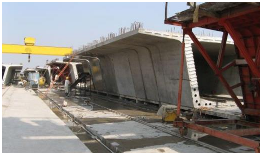
Figure 62 : Segments Casting in precast yard
