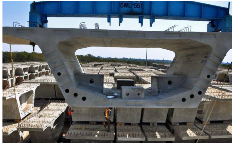
Figure 63 : Segments Stacking in precast yard
