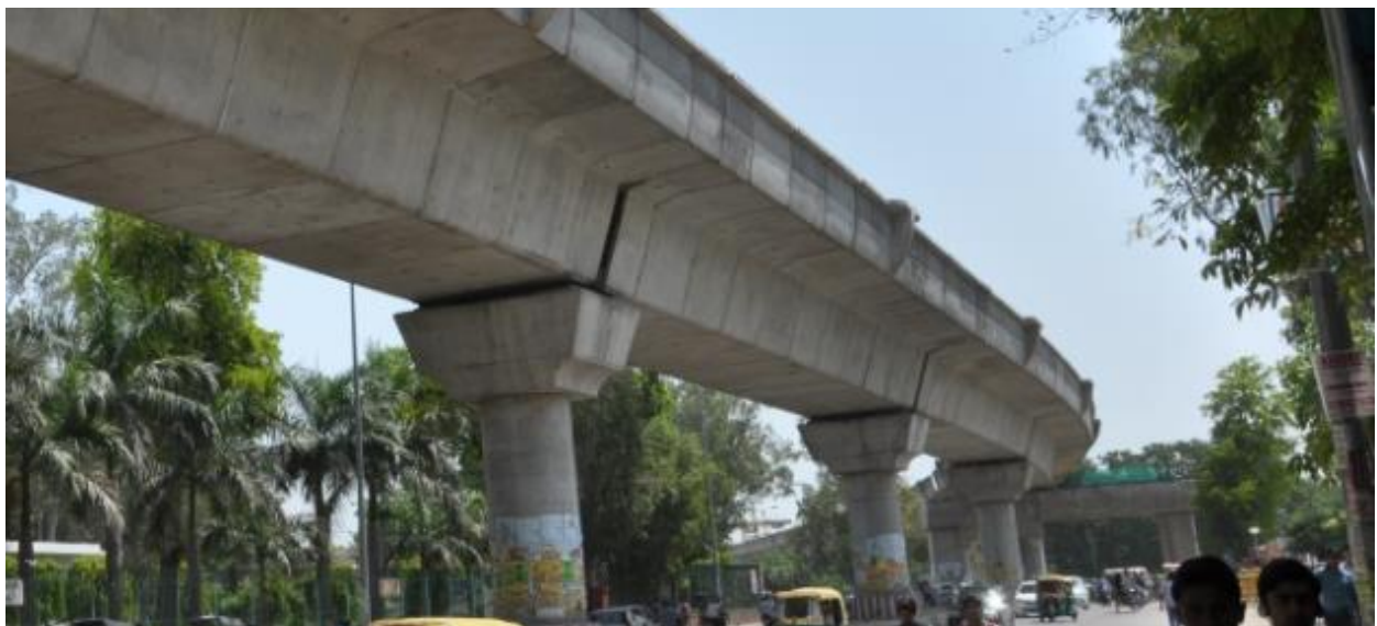
Figure 59 : RC Pier cap for Segmental Box-Girder Viaduct
