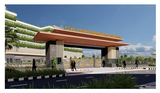
The Civil Court gate is designed as a focal point to direct the commuters to the stations. Conceptually it is a grand entry and architecturally it is a contextual modern design depicting the grandness of the station. The design element has been taken from the station i.e use of Basalt stone and GRC Jali for the gate design.
