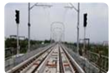
Signalling Outdoor Signal Installation work
